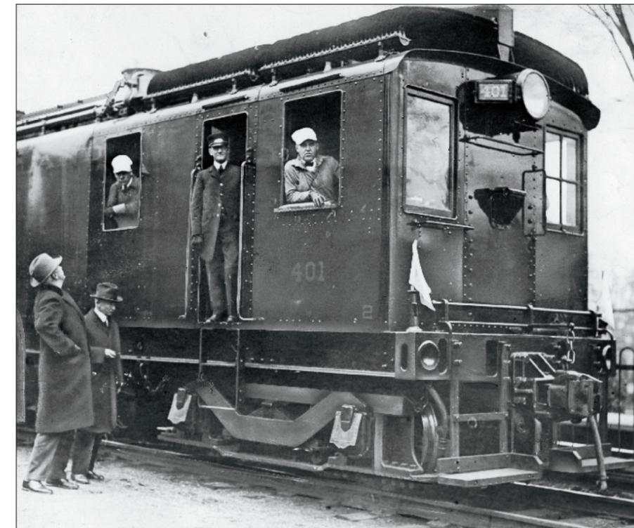
**Long Island Rail Road No. 401, a 100-ton boxcab built by Alco/GE/Ingersoll-Rand, is often credited with being the first road diesel-electric in the U.S. Long Island Rail Road**
