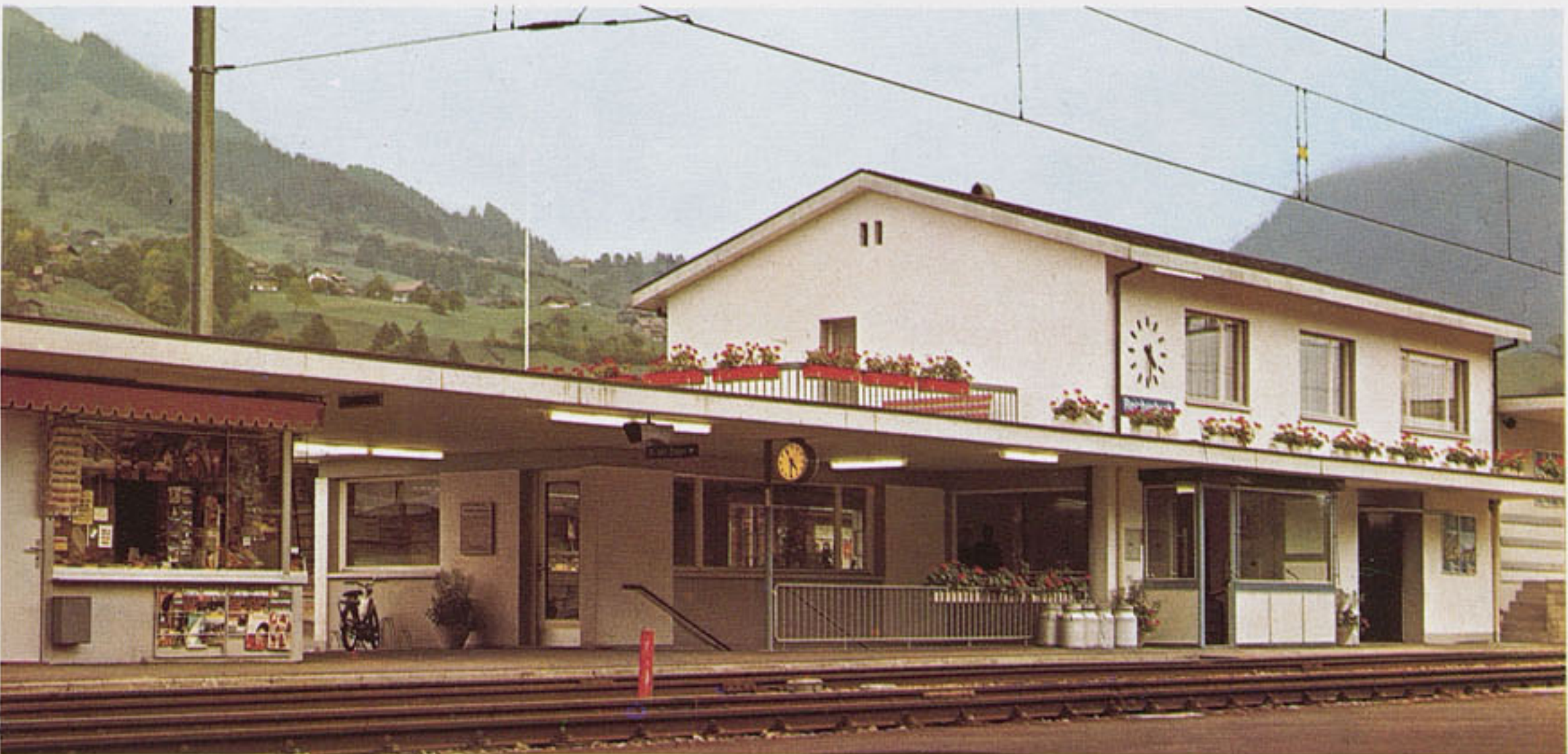
B 201 Bahnhof Reichenbach. Large modern type main line station. Gare Reichenbach. Stazione moderna Reichenbach.
