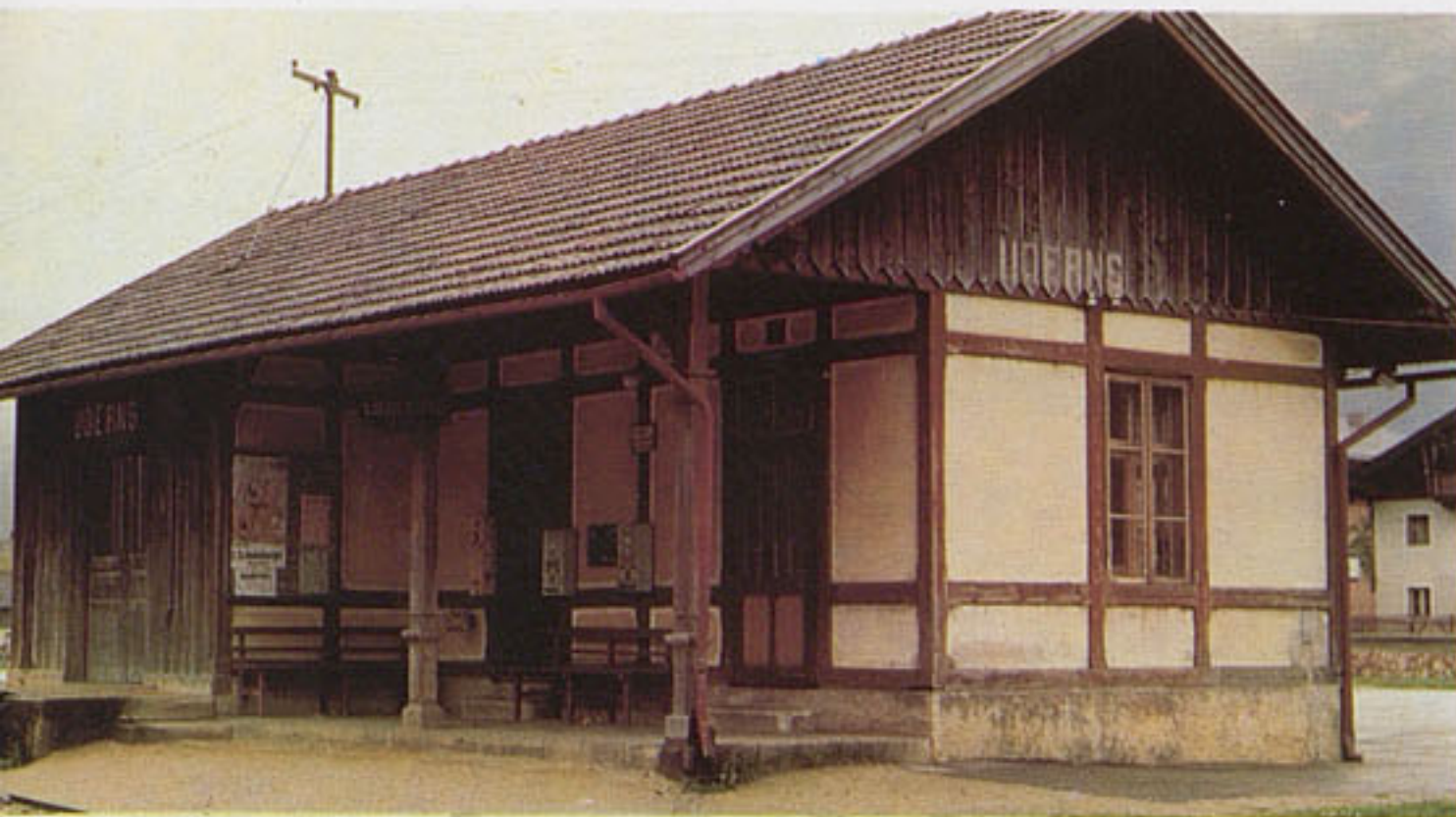
B 803 Station „Uderns“. Country styled station. Gare Uderns. Stazione Uderns.
