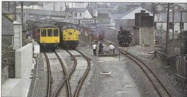
LEFT: At Blaenau Ffestiniog, North Wales, the standard gauge (4ft 8½in) tracks of British Rail and narrow gauge tracks (1ft 11½in) of the Ffestiniog Railway meet.
