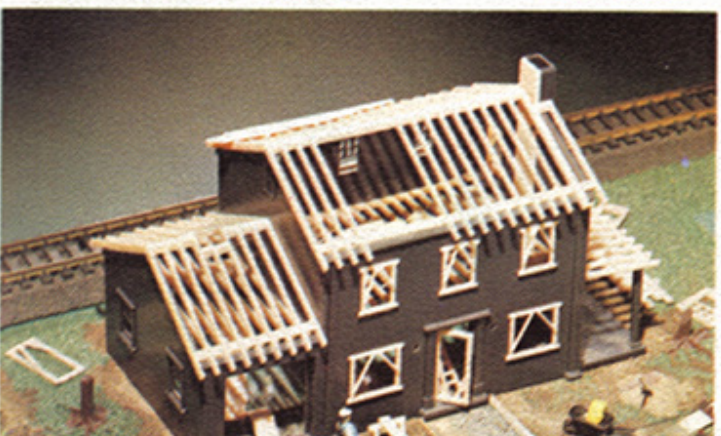
2803 HOUSE UNDER CONSTRUCTION
